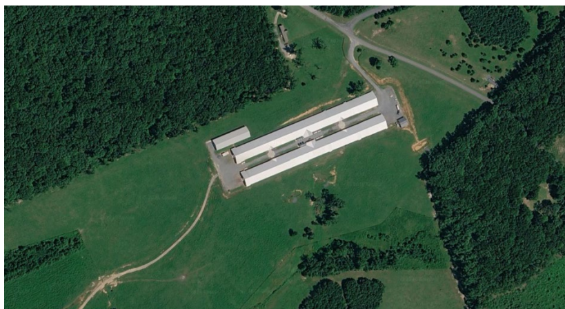
Example poultry facility with litter shed. Image Credit: Google Maps
