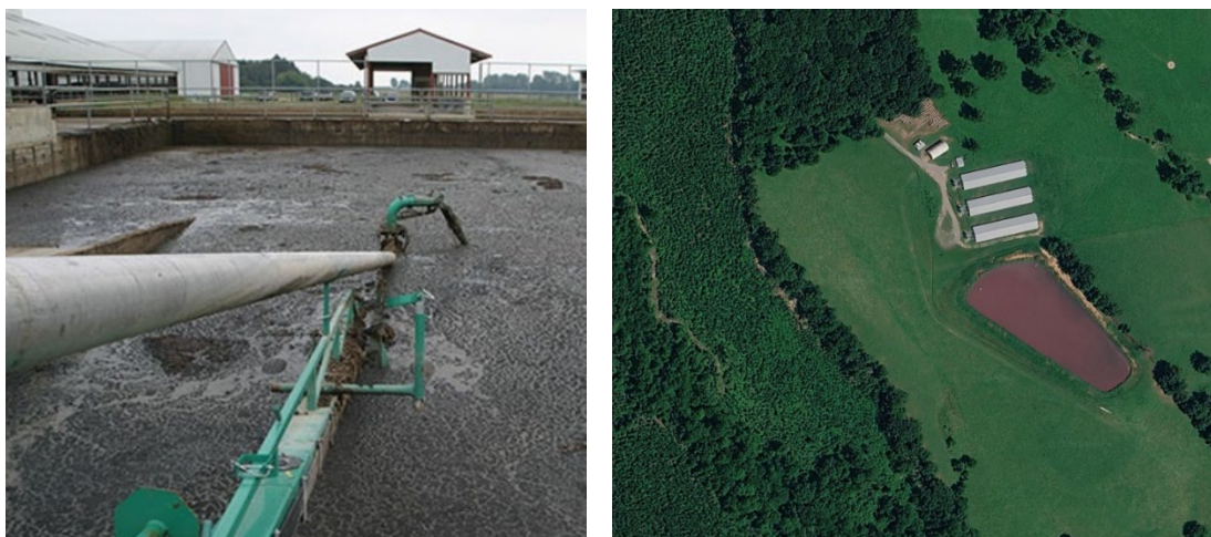
Example liquid manure storage pit (top left) and lagoon (top right). Image Credit: Virginia Tech Environmental Health and Safety (left); Google Maps (right)
